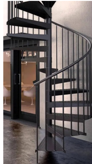
Metal spiral staircases in duplex roof dwellings (S.M.A.O.)
